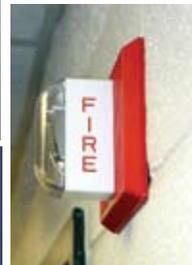
Speakers are automatically actuated by the fire alarm system in a fire event, and following a pre-alert tone, selected groups of speakers may transmit one or more prerecorded messages directing the occupants to safety. Trained personnel activating and speaking into a dedicated microphone can suppress the replay of automated messages in order to initiate or relay time voice instructions.
